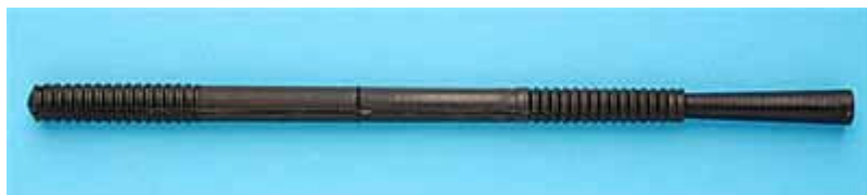
Fig.2. Holdfast remedial wall-tie. Top: as supplied to user, ready for insertion;
